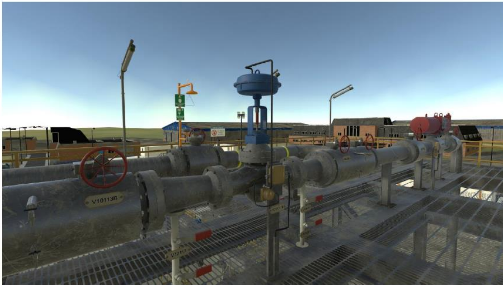
Figure 7 – Top of platform PCV with isolation, bypass and drain valves
