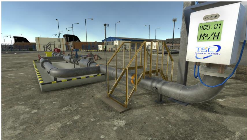
Figure 4 – Crude oil feed showing control valve and inlet flow controller
